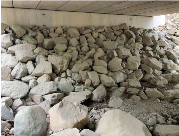
Left Bank Abutment when facing downstream
