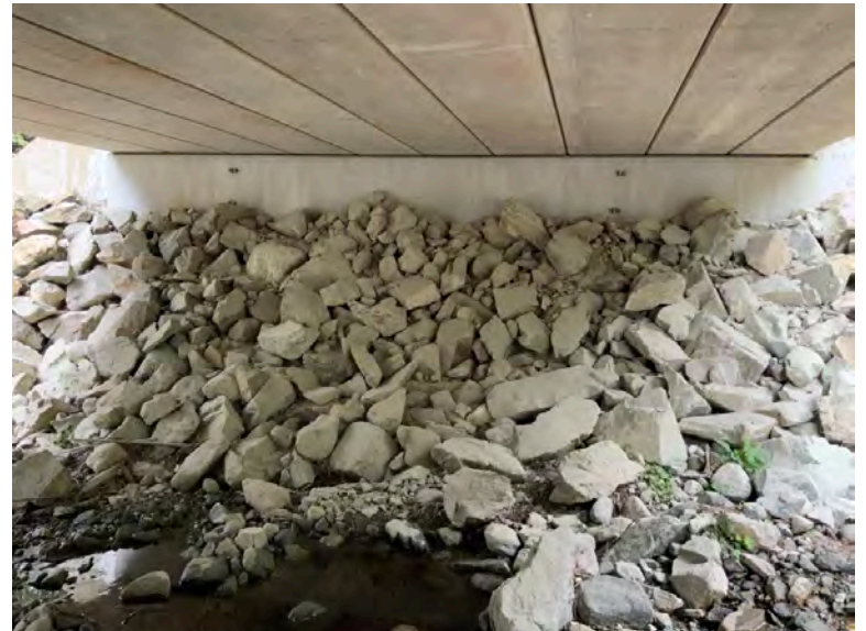
Right Bank Abutment when facing downstream
